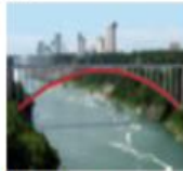
Bridge (red line) is unreachable because of underneath water flow
