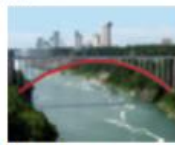
Bridge (red line) is unreachable because of underneath water flow
